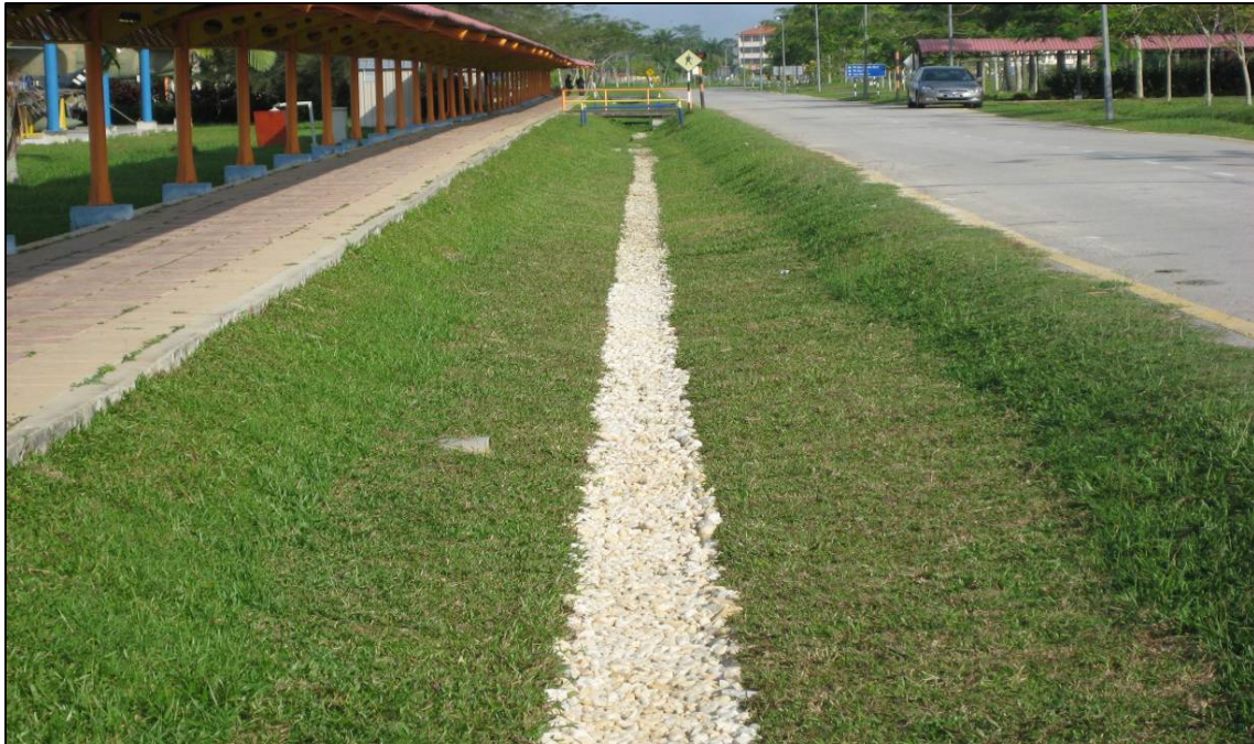
Figure 2. An ecological swale with river gravels making up the low flow channel.
