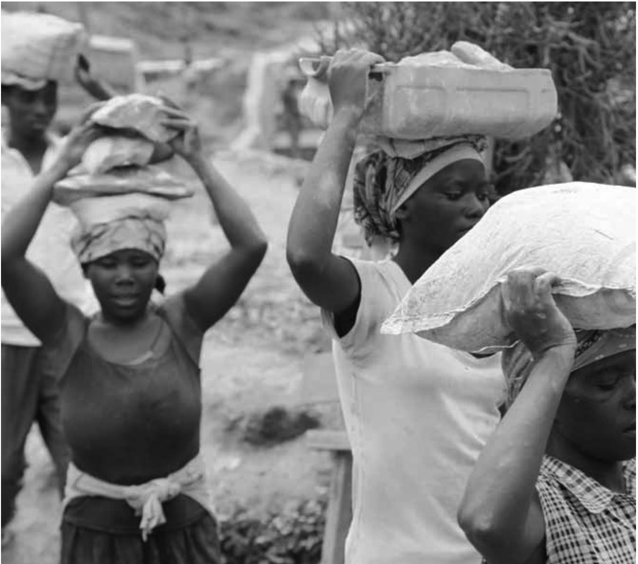
Ongoing construction of a water tunnel in Bugesera, Rwanda. © UN-Habitat/Julius Mwelu
