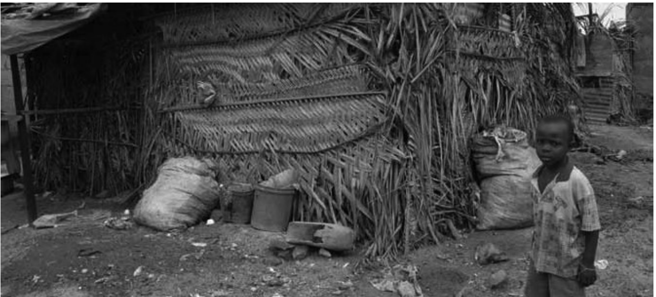
Fragile structures in Manzese, a densely populated neighbourhood in Dar Es Salaam, Tanzania.
