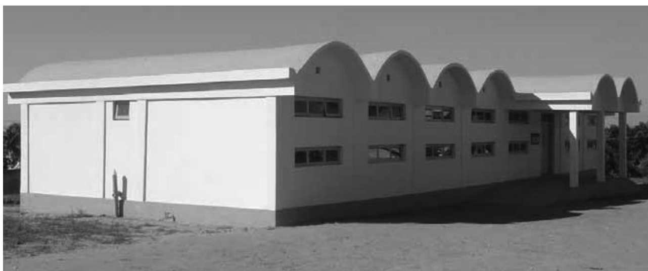
Cyclone-proof kindergarten in Vilankulo, Mozambique. © UN-Habitat/Arianna Francioni
