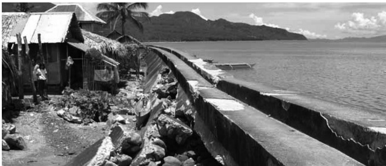
Seawall in Sorsogon City, Philippines © UN-Habitat/Bernhard Barth
