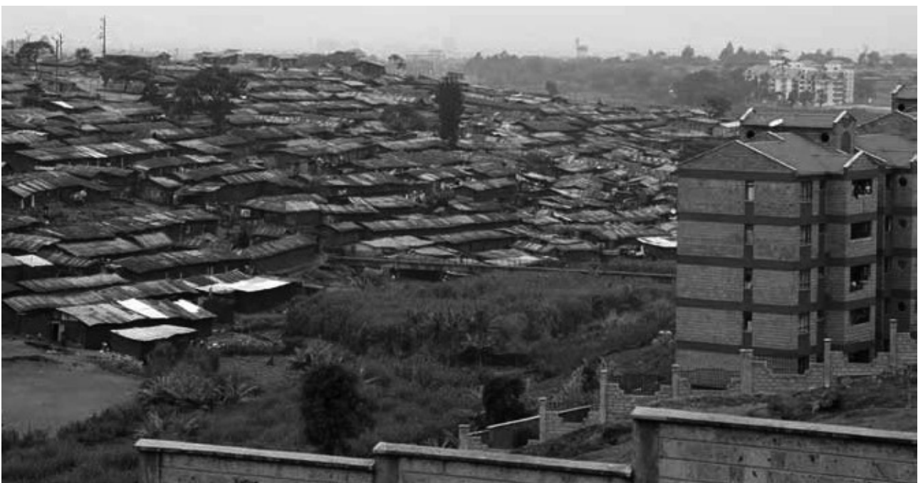
Newly constructed residential flats built as a rehabilitation settlement to relocate slum dwellers in Nairobi, Kenya.
