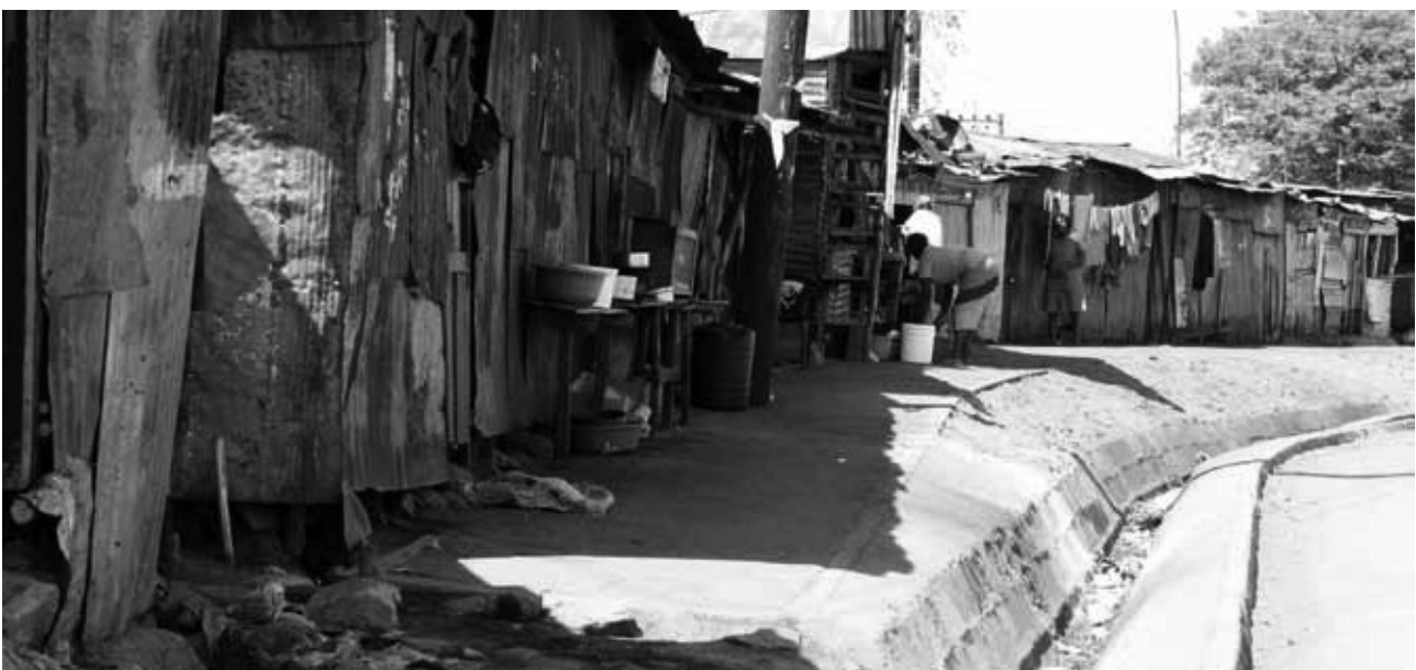
Newly constructed drainage, Kibera. © UN-Habitat/Bernhard Barth
