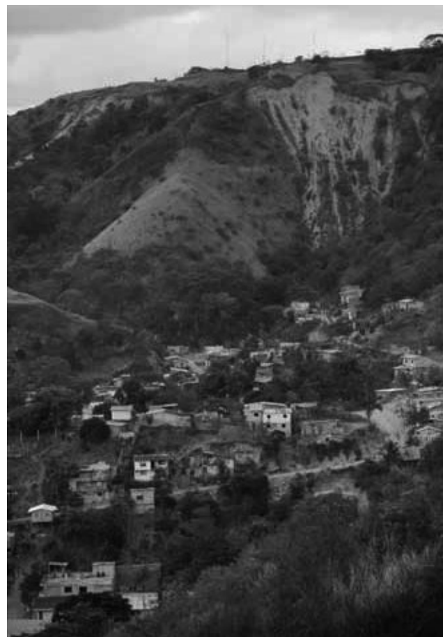
A landslide in Cerro del Barrio Lindo gatazo affects several houses built on hillsides in Esmeraldas, Ecuador.
