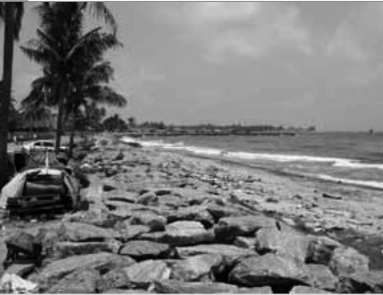
Negombo seawall. © UN-Habitat/Bernhard Barth
