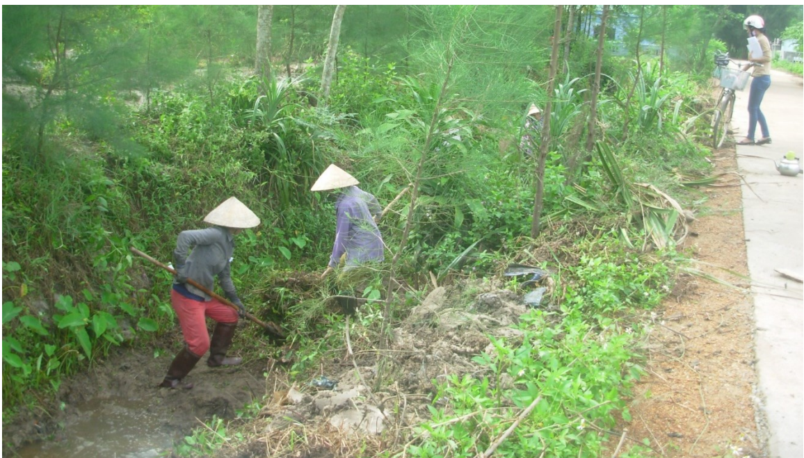
Figure 8-1: Dredging blocked drainages in June 2013
