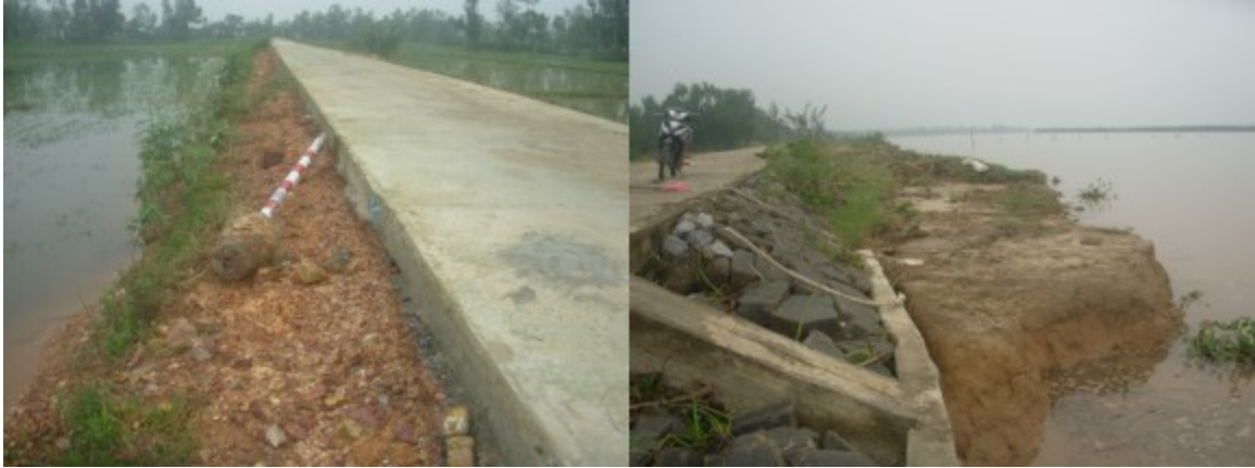
Figure 7-3: Emergency road and dyke in Lang eroded by floods and tidal flooding in 2013
