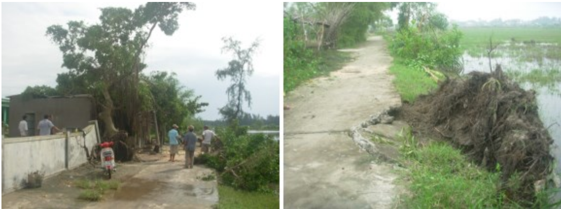
Figure 7-2: Damage to a house and a road during the storm in September 2013
